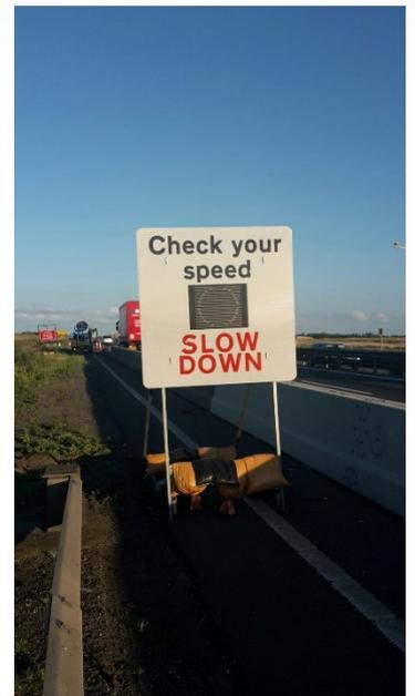
Radar speed sign technology is a successful technique being used for traffic calming efforts. These signs are proven to help reduce drivers' speeds in both the short and long term. Morelock's radar speed signs equipped with software that capture driver speed and relevant traffic data have been deployed in a host of applications from small communities to larger industrial sites and in partnership with the police force to tackle speeding by educating and changing driver behaviour.
